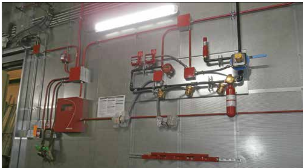
The final fire suppression system for the diesel gensets is pictured here.
